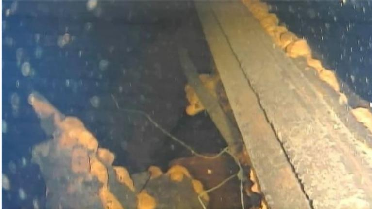
Figure 1.1: Picture of possible melted nuclear fuel inside the Fukushima nuclear plant [1].
