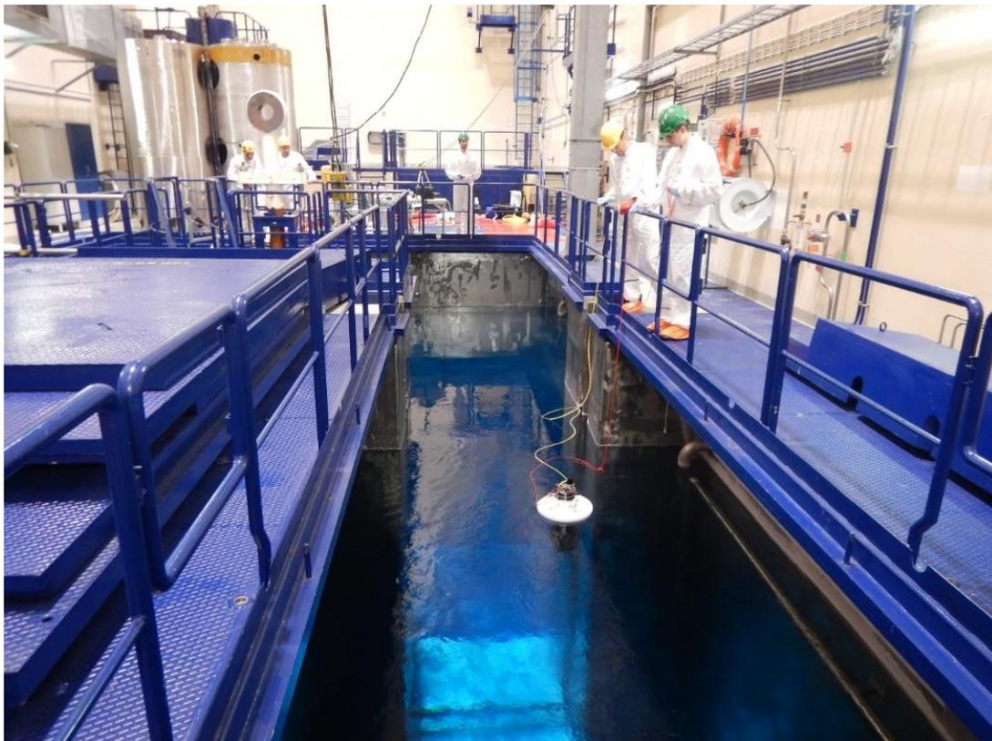
**Figure 4** USV Datastart deployed in the interim spent fuel storage pond. Note the walking bridge over the water, preventing a proper alignment of ICVD or using SFAT when performing verification close to the walls. The USV could navigate below the bridge.
