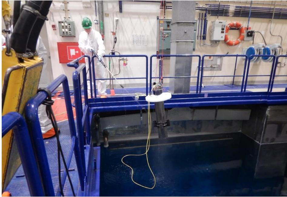
**Figure 1** Cleaning procedure - jet-washing over the pond; the system was wiped dry afterwards. The overhead crane, operated by the facility staff, was used for putting the USV in and retrieving it out of the storage pond.
